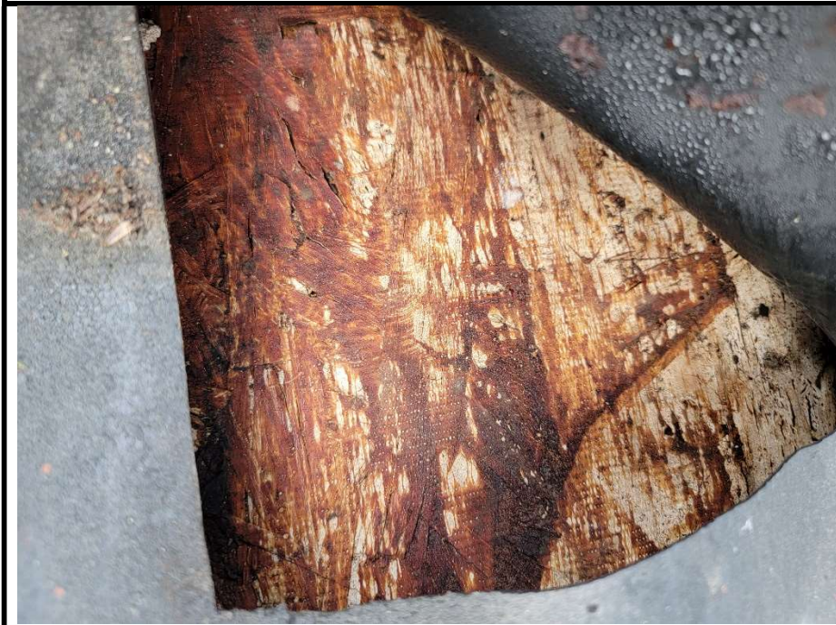
27. 234 Roof – Assumed ACM White Membrane and materials below
