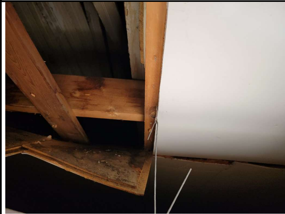
19. 234 – Non-Suspect Cellulose Ceiling Tiles found above 2'x4' P'n'F Ceiling Tiles
