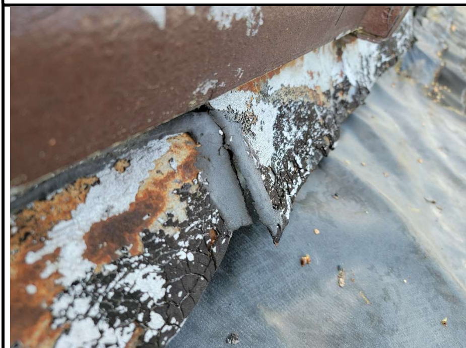
26. 234 Roof – ACM Silver/Aluminum Paint at Parapet
