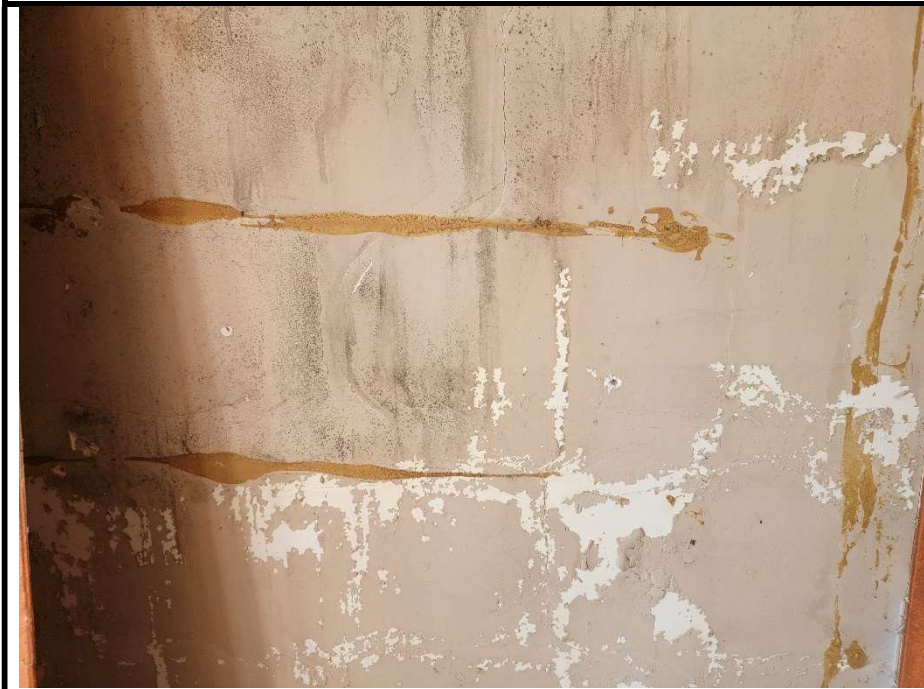
15. 240 – Non-ACM Paneling Glue on Wall
