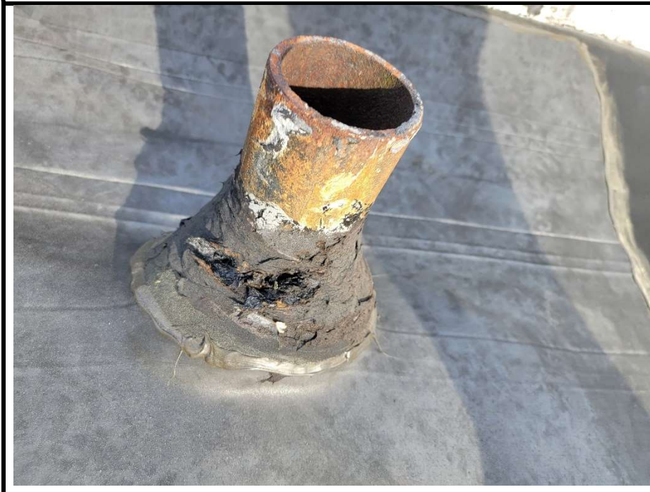
28. 234 Roof – Non-ACM Black Asphalt Mastic at Intrusions
