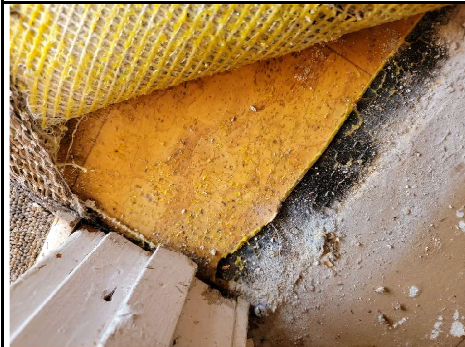
14. 240 Front Room – Carpet over Non-ACM Yellow Vinyl Sheet Flooring
