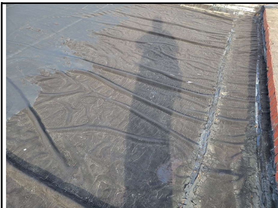
25. 234 Roof Membrane – Non-ACM Black Asphalt Mastic
