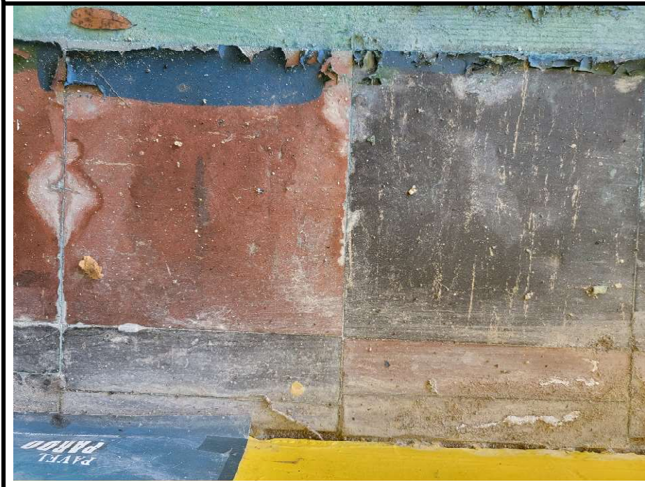
4. 236 Main Room – ACM 9"x9" Red with White Streaks Vinyl Floor Tile and ACM 9"x9" Black with White Streaks Vinyl Floor Tile
