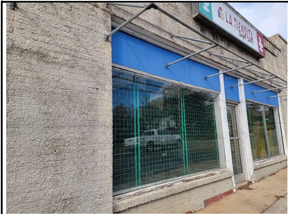
17. 236 Front Façade with Non-ACM Siding Coating
