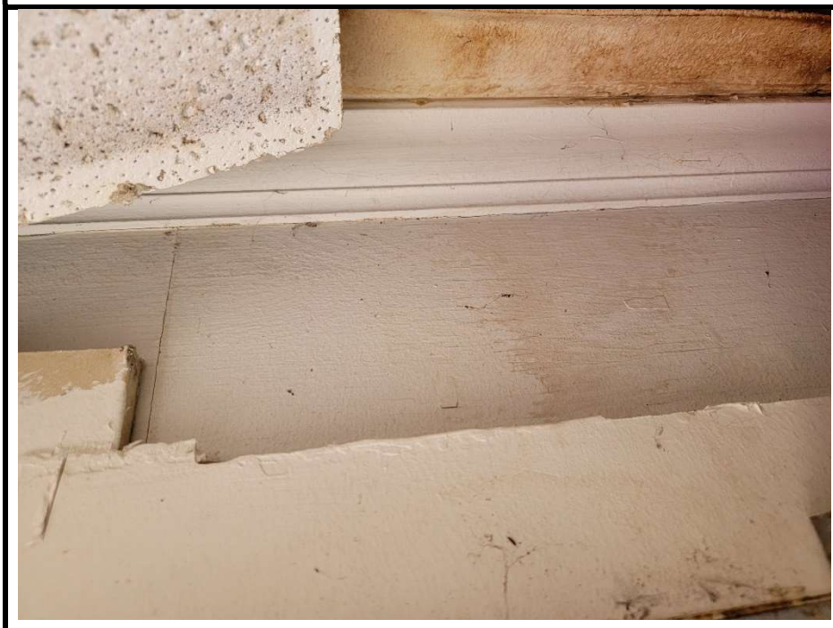
18. 234 – Non-ACM Plaster Wall behind Non-ACM Drywall/Joint Compound Walls and Non-ACM 2'x4' P'n'F Ceiling Tile
