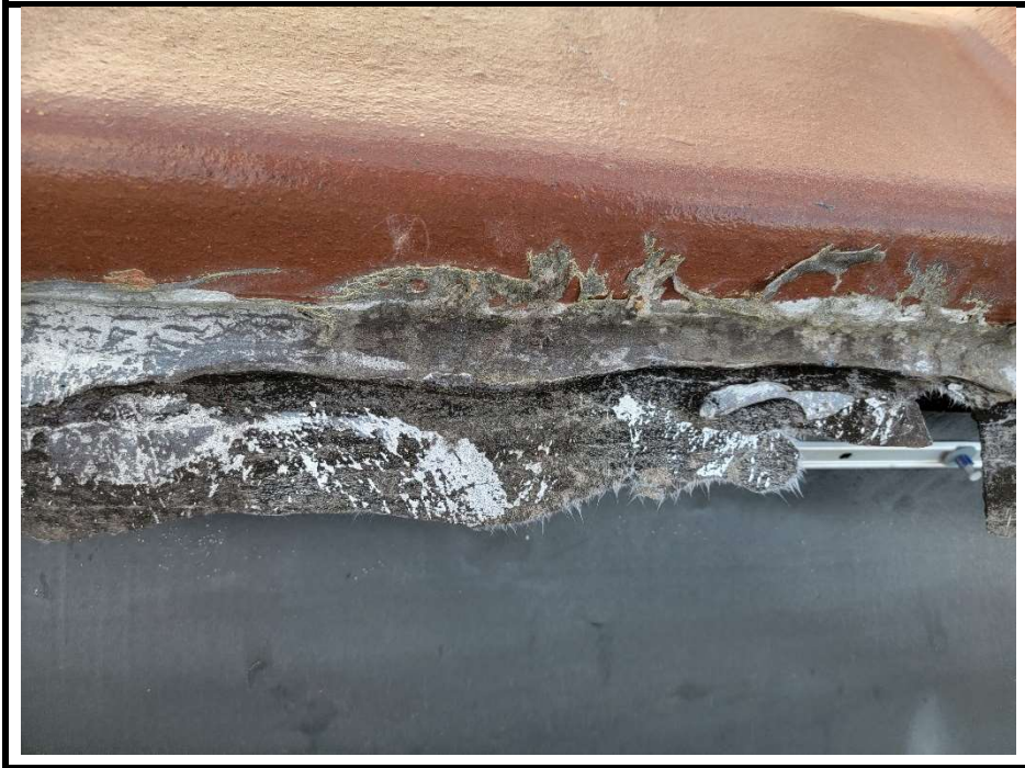
29. 234 Roof – ACM Silver/Gray Caulking at Front Parapet
